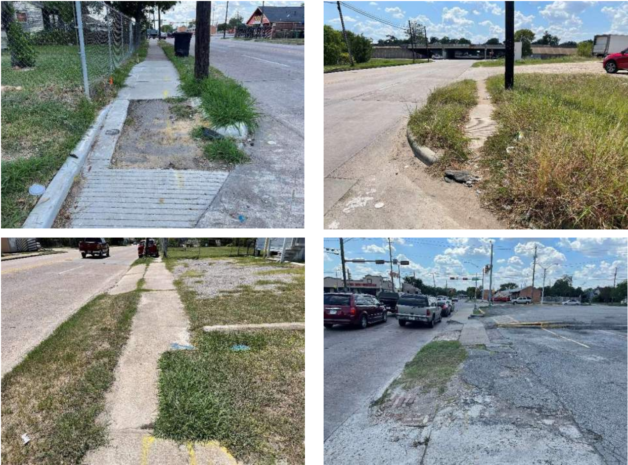
Figure 3.3 Patton Street Existing Sidewalk and Ramp
