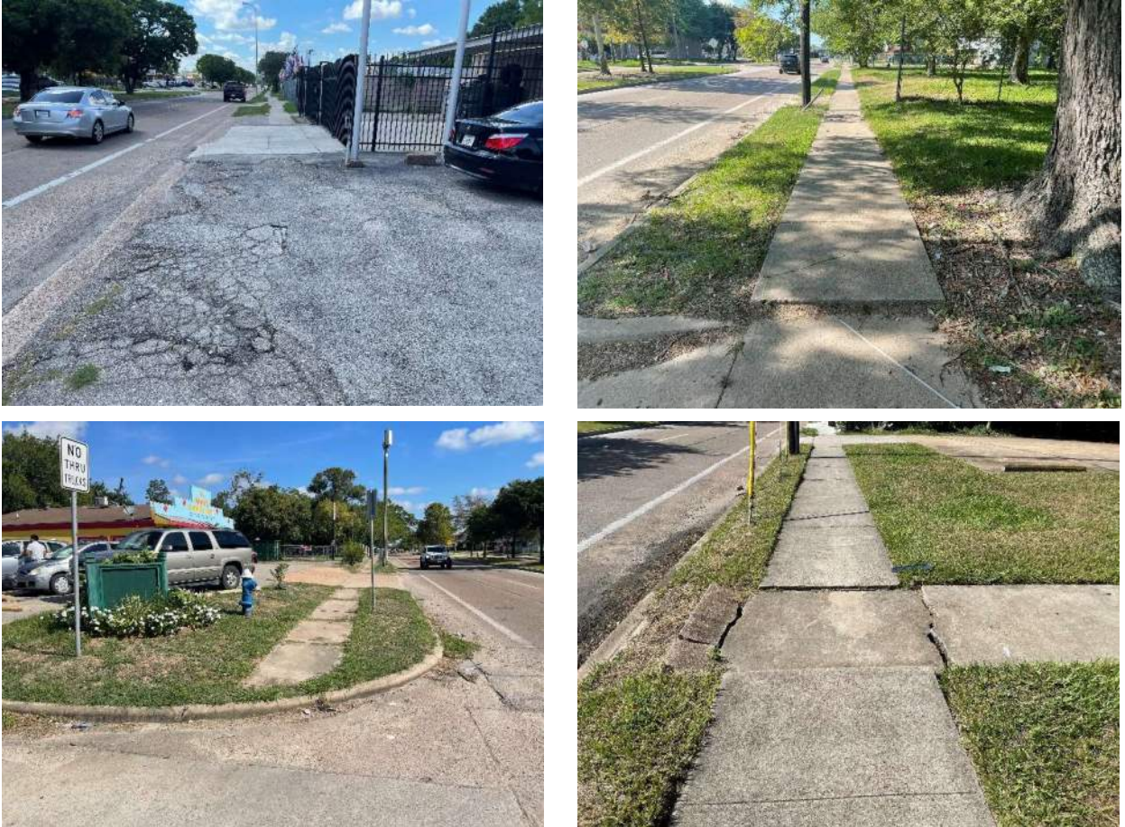
Figure 3.6 Irvington Blvd Existing Sidewalk and Ramp
