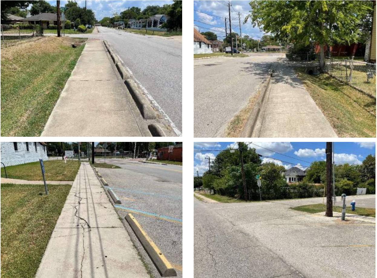
Figure 3.4 Link Road Existing Sidewalk and Ramp
