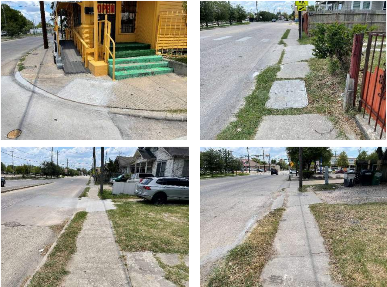
Figure 3.2 Fulton Street Existing Sidewalk and Ramp
