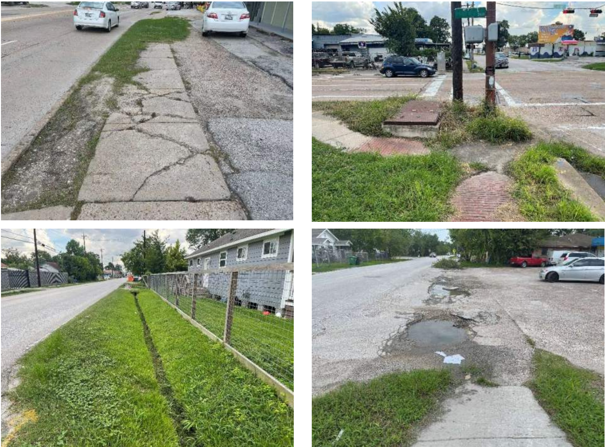
Figure 3.8 Collingsworth Street Existing Sidewalk and Ramp
