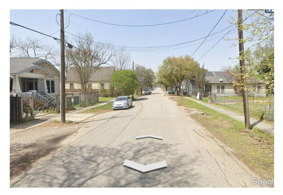
Fulton Street at Burnett Street Existing Conditions: No curb or gutter +/- 25 foot Roadway Cross Section
