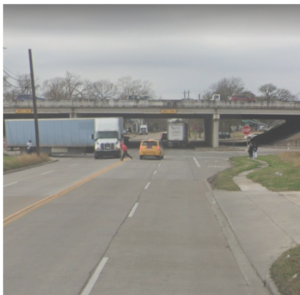
Overgrown and narrow sidewalks along Patton Street looking toward I-45.
