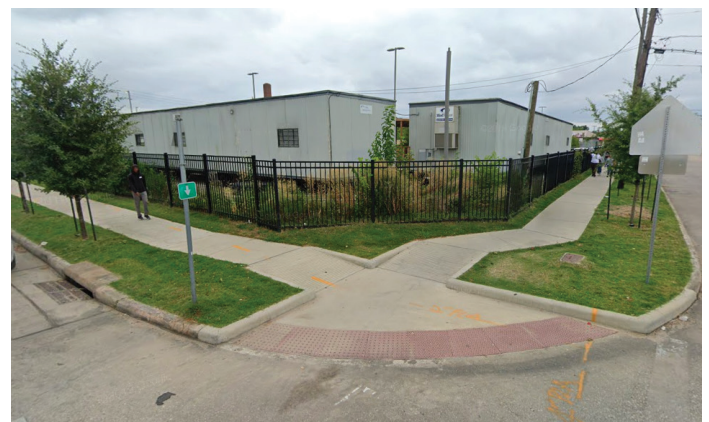
Newly improved sidewalks, at Fulton St and Morris St feature paths at least six feet in width and accessible ramps. Map Data: 2019 Google
