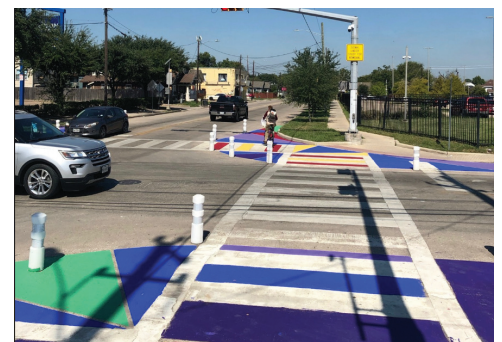
Recent Quitman Street at Fulton Street intersection improvements TIRZ 21 Mobility Recommendations
