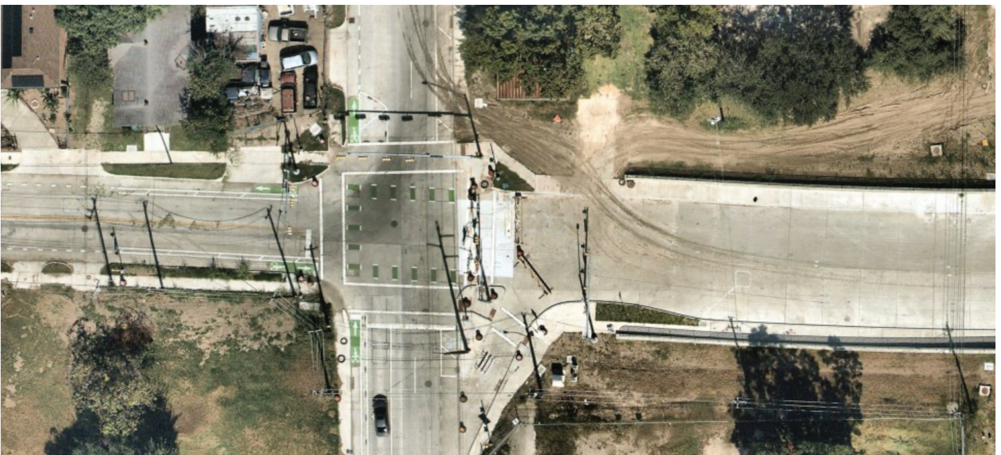
Lorraine Street at Hardy Street with bike lane intersection markings and connections to the newly constructed railroad underpass to the east. Example of connectivity for other corridors.
