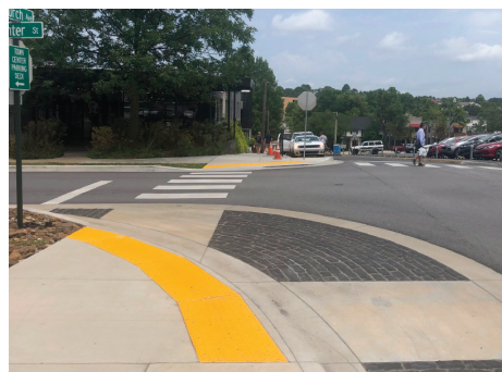
Permanent intersection improvements from tactical urbanism-project in Fayetteville, AR
